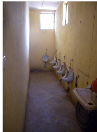
Ph. 17: Latrine 1 (int.)
