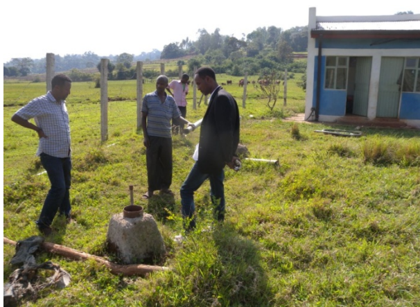
Ph. 6: Borehole BH1 burned by lightning
