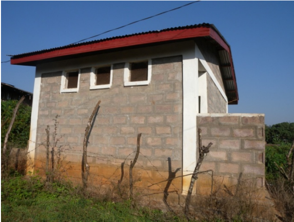
Ph. 17: Latrine at the Bus station
