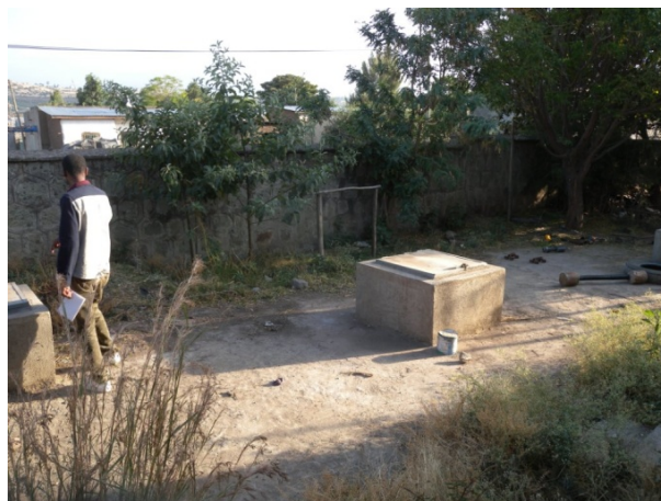
Ph. 33: Toilet septic tank
