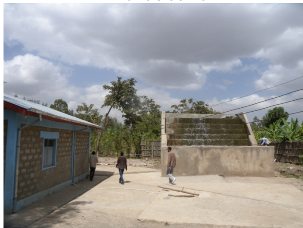
Ph. 12: Makane Booster, step aerator and water reservoir
