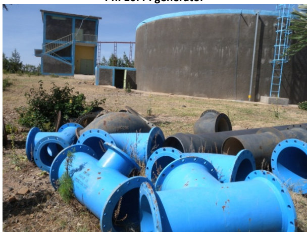
Ph. 12: new water Tank
