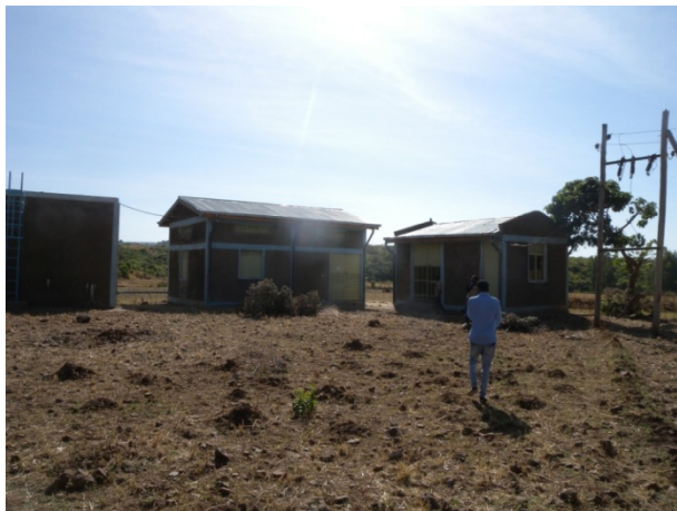
Ph. 8: Booster buildings
