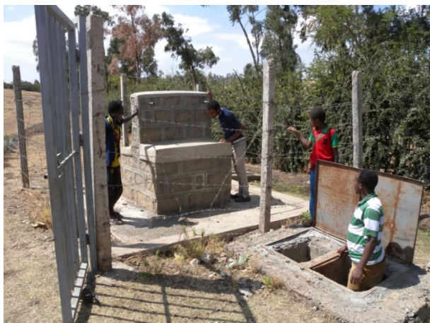
Ph. 27: Water point n. 1 (out of service)
