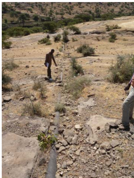
Ph. 21: Transmission pipe, not buried
