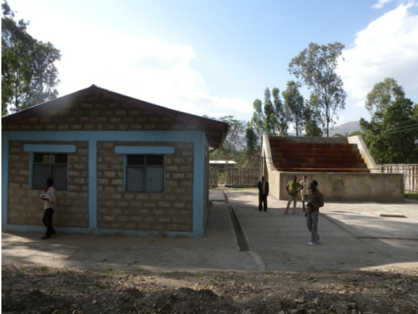
Ph. 19: Benara Booster2, step areator and wet tank
