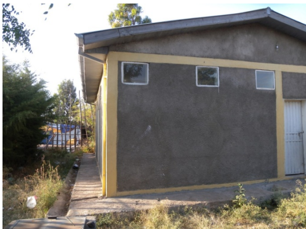
Ph. 32: Toilet at the bus station/market
