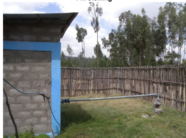
Ph. 8: Borehole BH1
