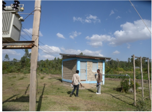
Ph. 18: Borehole BH2 at Benara site
