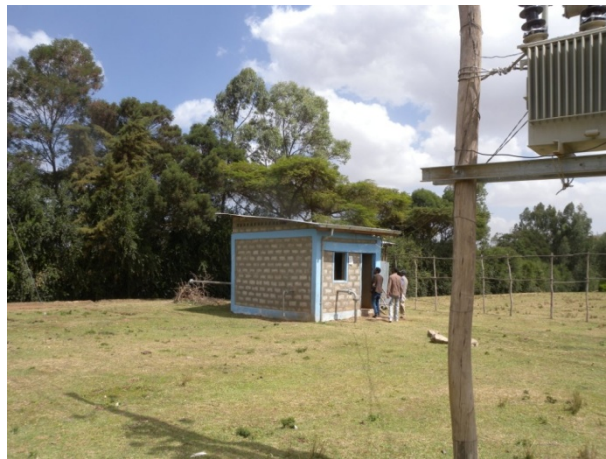
Ph. 10: Borehole BH3
