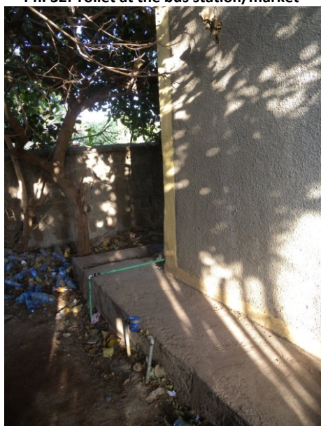
Ph. 34: Toilet Water connection
